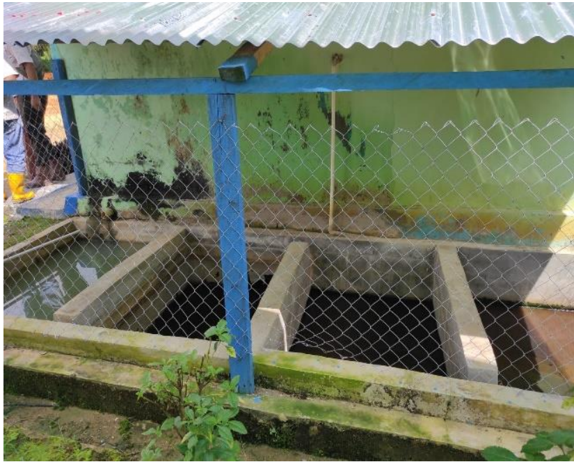
Photo 7: Settling pond of equipment washwater (PT BAS)
