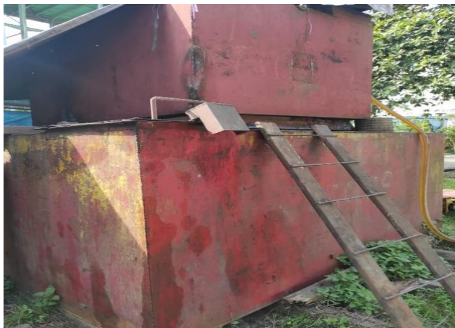
Photo 6: Diesel Oil Above Storage Tank, without secondary containment or appropriate signage (PT SWA)
