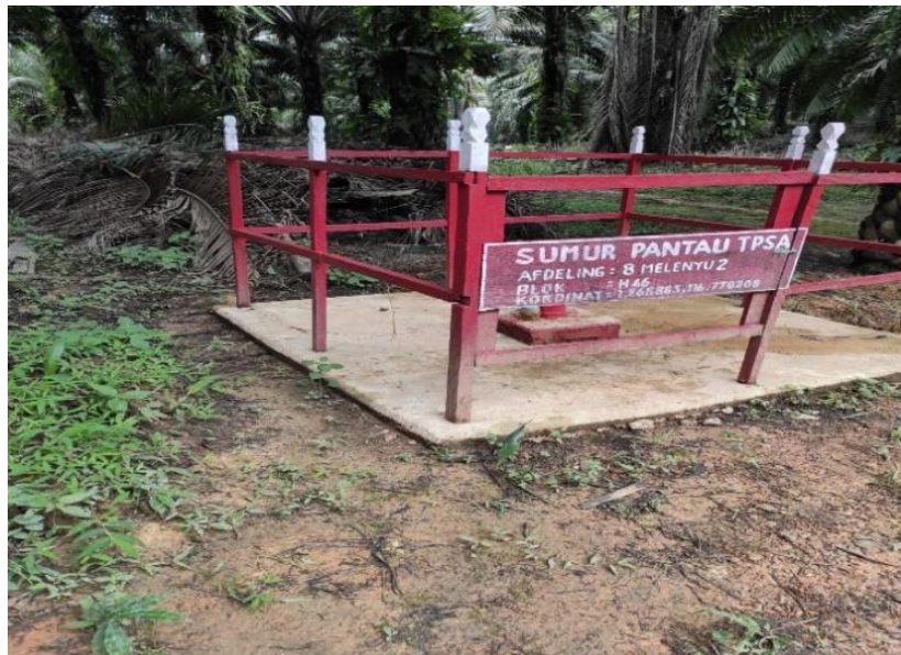
Photo 4: Groundwater monitoring well adjacent to on-site landfill site (PT DWT)
