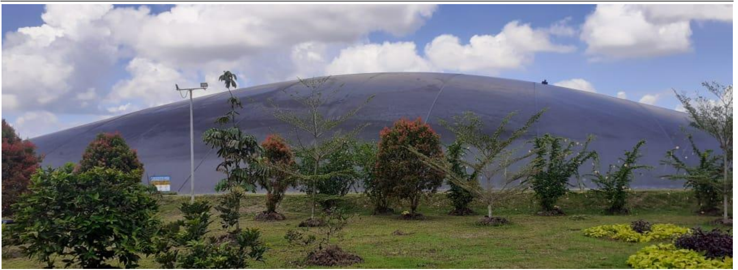
Exhibit 13. Bio-CNG plant dome
